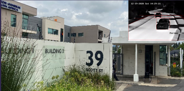
Office building entrance
